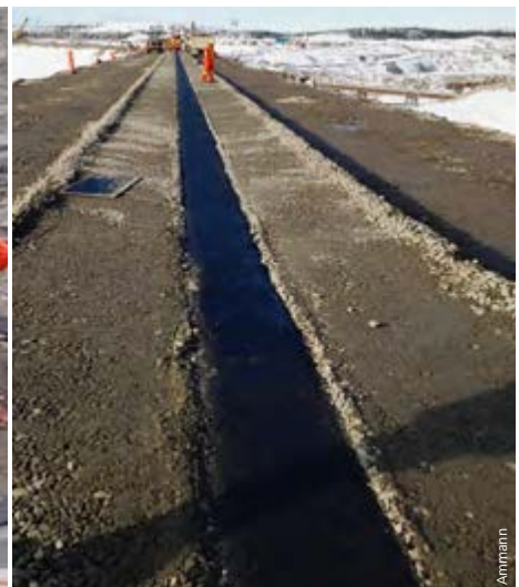
The asphalt core is built up layer by layer over the entire length of the dam.
