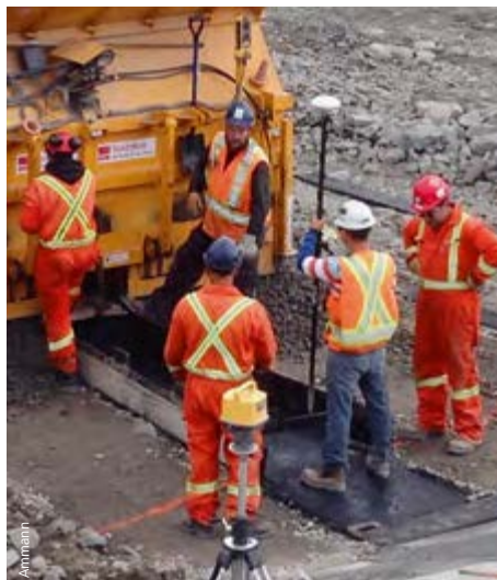
The asphalt core is built up layer by layer over the entire length of the dam.
